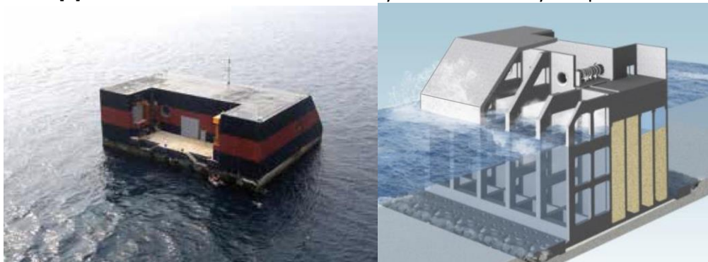
Figure 7 – Nearshore bottom-standing OWC system Yongsoo plant, South Korea [6]
