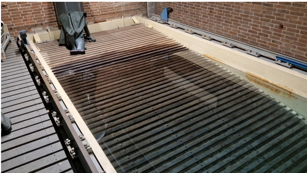
Figure 15: Wave damping beach of towing tank number 2.
