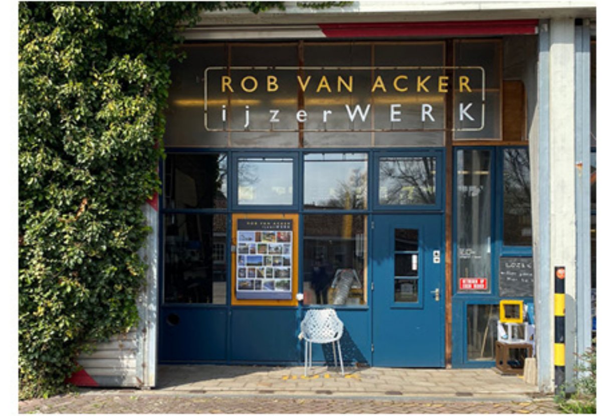
individual front facades
