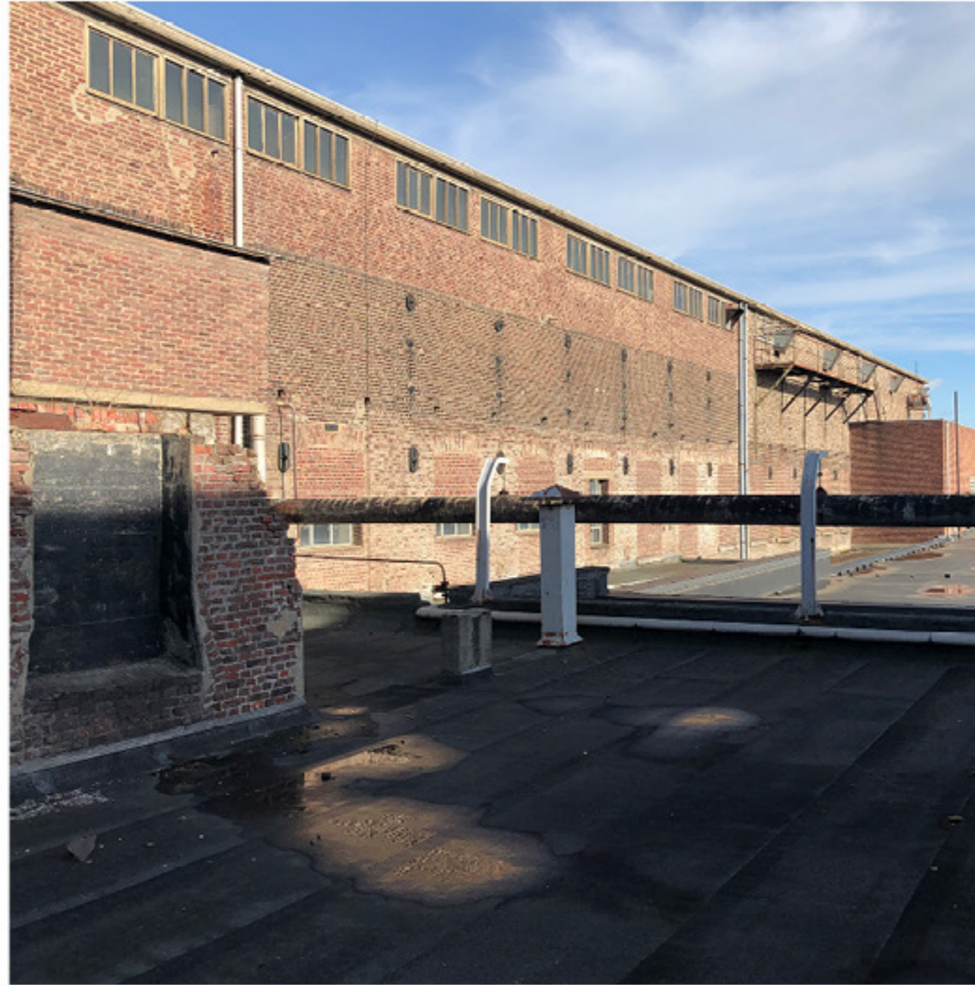
existing south facade
