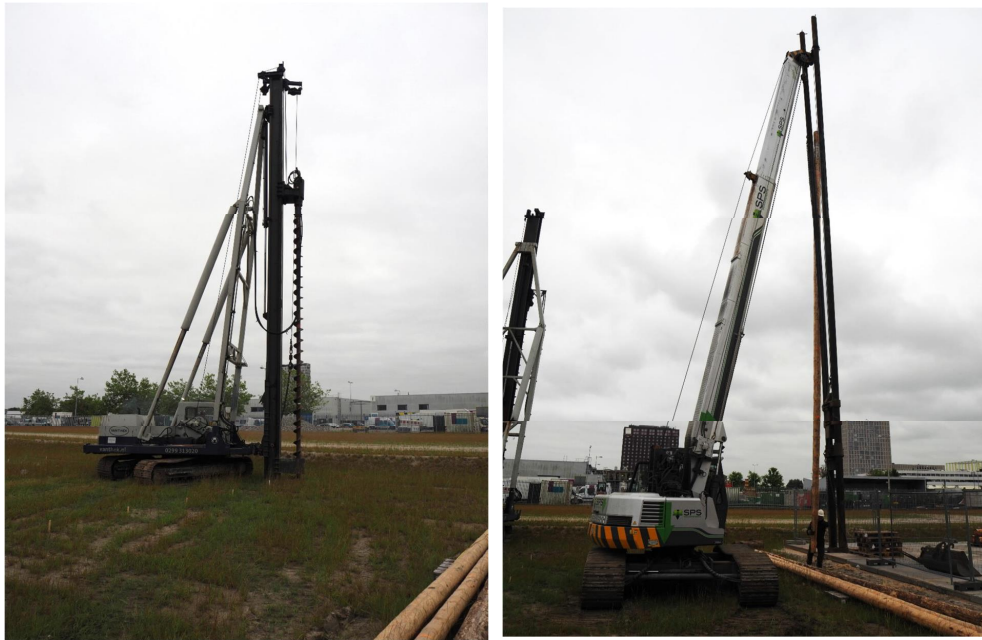
Figure E.5: Preparation: Soil Pre-drilling (left) and Pile Installation (right)
