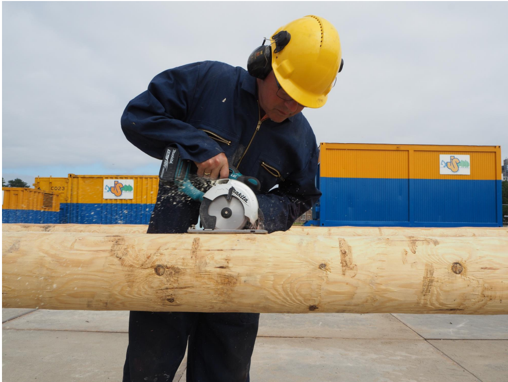
Figure E.3: Preparation: Sawing grooves for fiber installation
