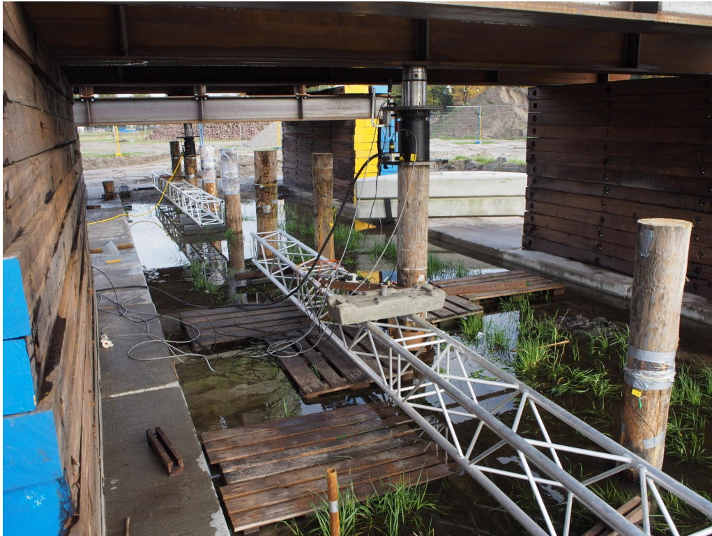
Figure E.7: Installed Piles with Load Cell and LVDT's
