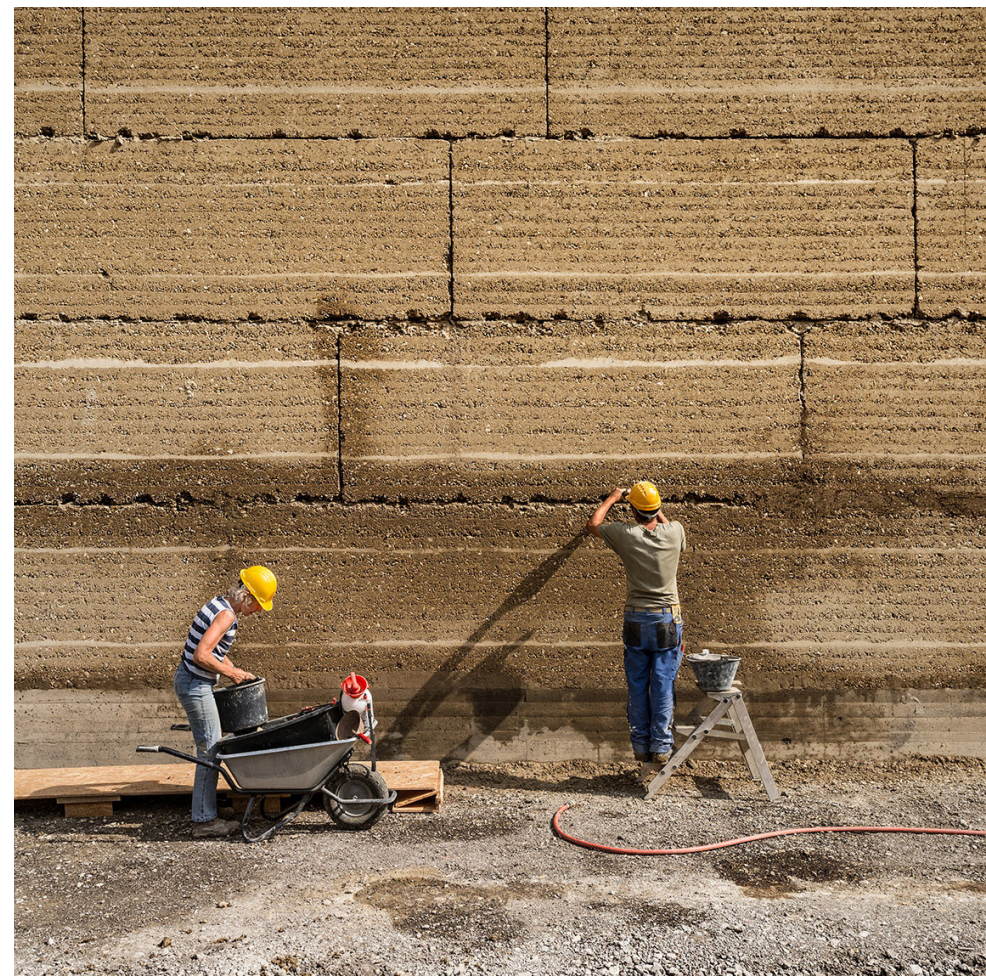
Collective Production of Space / Rammed Earth Walls © Iwan Baan
