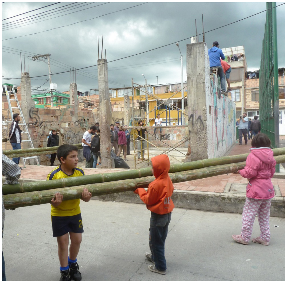
Collective Production of Space © Arquitectura Expandida
