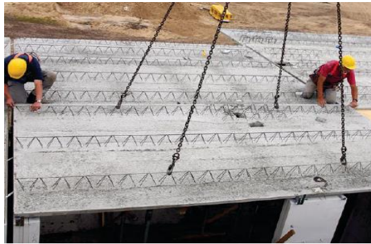
(a) Reinforced plank floor without concrete topping [88]
