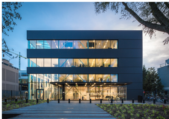
(a) The Temporary Courthouse Building
