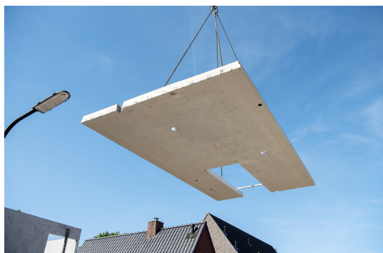
(a) Bestcon floor slab with integrated recess [93]
