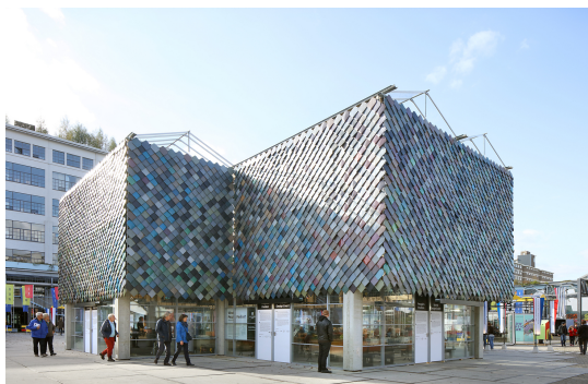
(a) Building overview
