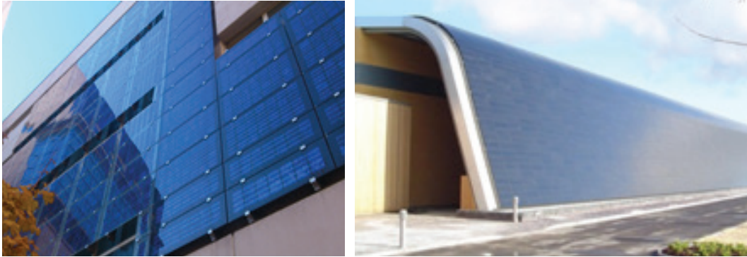
FIGURE A.3: EXAMPLES OF COMMERCIAL BUILDINGS OR HOMES WITH INTEGRATED FLEXIBLE SOLAR PANELS INTO THEIR ARCHITECTURE. LEFT IMAGE: PHOTOVOLTAIC SOLAR FACADE ON THE MUNICIPAL BUILDING OF SOCIAL SERVICES CENTRE JOSE VILLARREAL, IN MADRID (SPAIN, 2013). SOURCE: COMMONS WIKIMEDIA, 2015. RIGHT IMAGE: APPLICATION OF FLEXIBLE SOLAR PANELS IN A BUILDING'S FACADE BY GSHK SOLAR TECHNOLOGY, 2011. SOURCE: GSHK, 2011.
