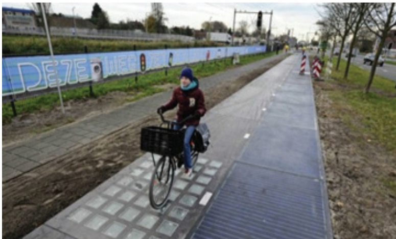
FIGURE A.19: "SOLARoad" BIKE PATH IN THE NETHERLANDS (2009-2014), IS MADE OF CONCRETE MODULES WITH DIMENSIONS 2.5 BY 3.5 METERS, EMBEDDED WITH SOLAR PANELS COVERED IN TEMPERED GLASS. THE SOLAR CELLS AT THE MOMENT PUT THE ELECTRICITY THEY GENERATE ONTO THE NATIONAL GRID, BUT FUTURE PLANS INCLUDE USING THE ENERGY TO POWER STREETLIGHTS. SOURCE: RTE, 2014.
