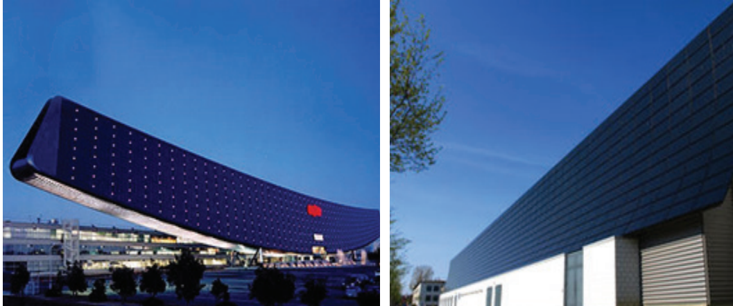
FIGURE A.1: LEFT IMAGE: SOLAR ARK IS A PV-POWERED BUILDING LOCATED NEXT TO SANYO'S SEMICONDUCTOR FACTORY IN GIFU, JAPAN. IT IS MADE BY MONOCRYSTALLINE SOLAR CELLS. THE CONSTRUCTION WAS ESTABLISHED IN DECEMBER 2001. SOURCE: INHABITAT, 2015. RIGHT IMAGE: FERDINAND-BRAUN-INSTITUT FÜR HÖCHSTFREQUENZTECHNIK IS A RESEARCH AND EDUCATION CENTER, LOCATED AT BERLIN ADLERSHOF IN DEUTSCHLAND. THE ARCHITECT CHRISTIAN MATZKE DESIGNS IT IN 2008. SOURCE: ARCHINOAH, 2015.
