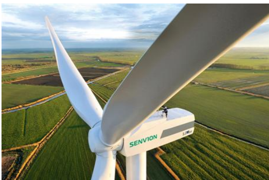
Figure 1: Senvion 3.2M114 Wind Turbine.
