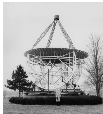
(c) Grote Reber and the first parabolic dish telescope (1937).
