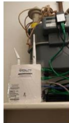
Figure 4.3: Electricity smart meter sensor mounted on a new digital meter (left) and an old gas meter (right). (Source: Monicair report)
