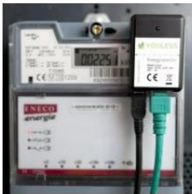
Figure 4.3: Electricity smart meter sensor mounted on a new digital meter (left) and an old gas meter (right). (Source: Monicair report)
