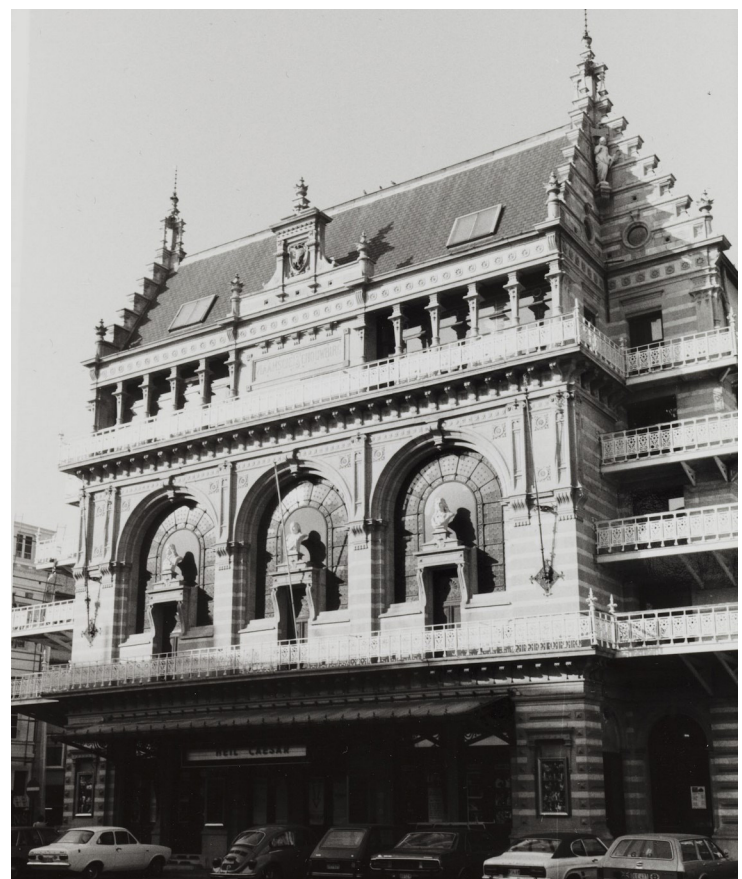
Figure 38: Flemish theatre, Rue de Laeken 146, Brussels
