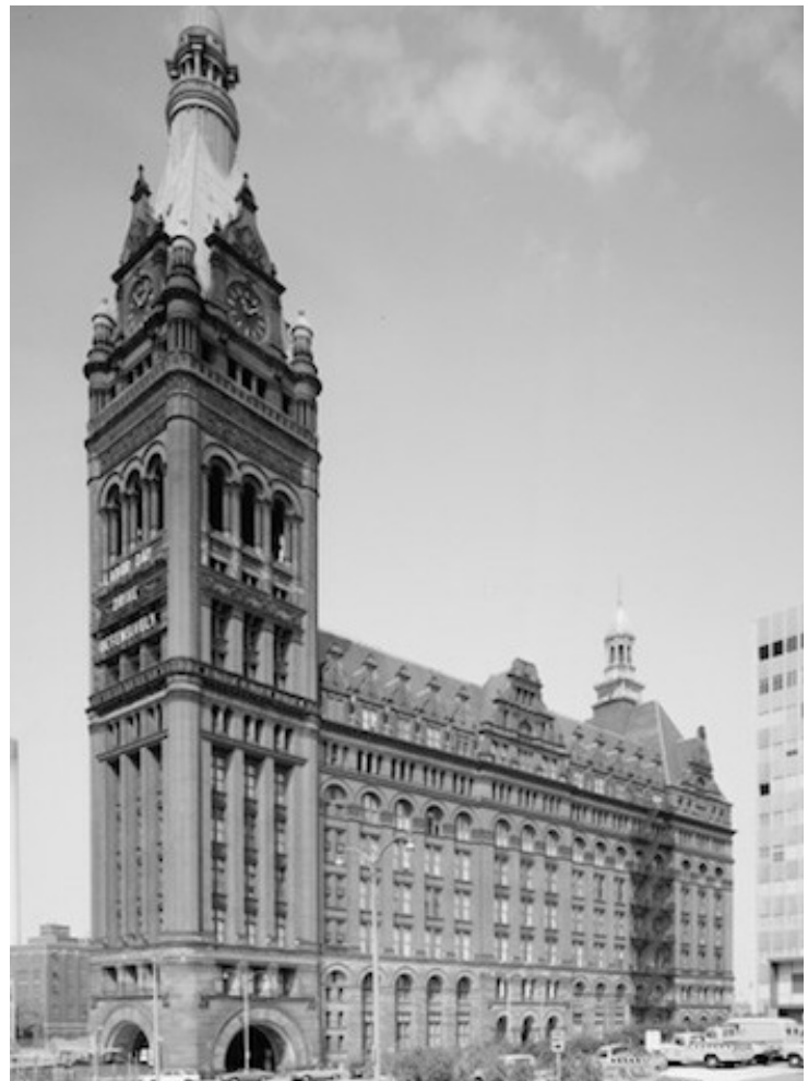
Figure 49. City Hall, Wisconsin avenue 1895
