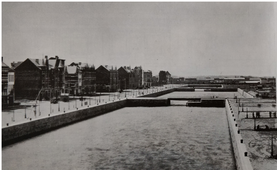
Figure 30: view of the Vlaamsekaai and the docks. 1879
