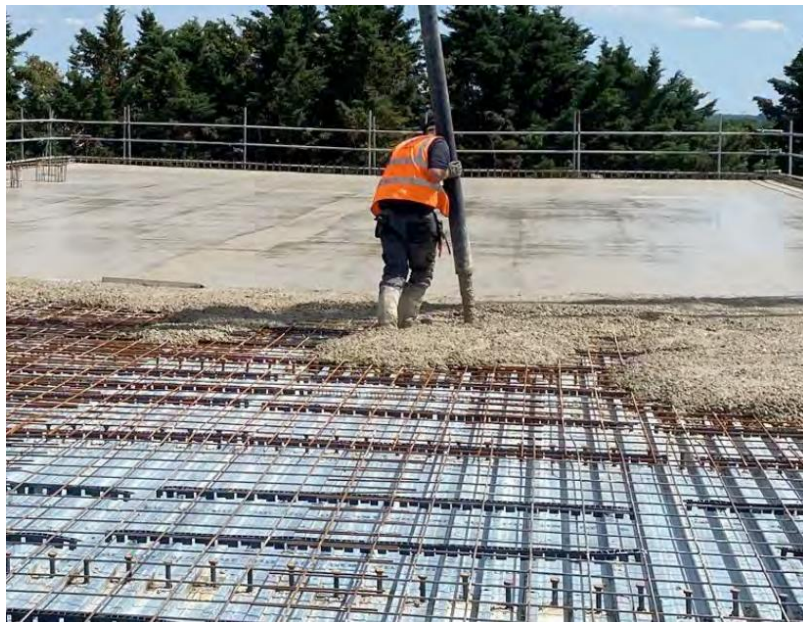
Figure 2.4. Concrete poured onto the steel sheeting [1].
