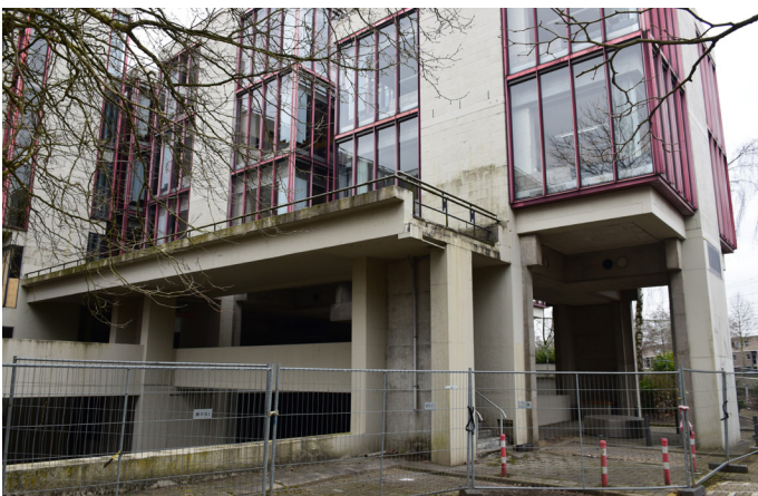
Fig. 15: South-west street enclosure.
