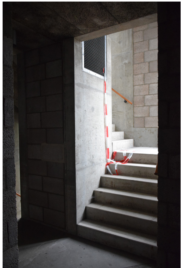
Fig. 172: Stairwell located at the four ends of the street.
