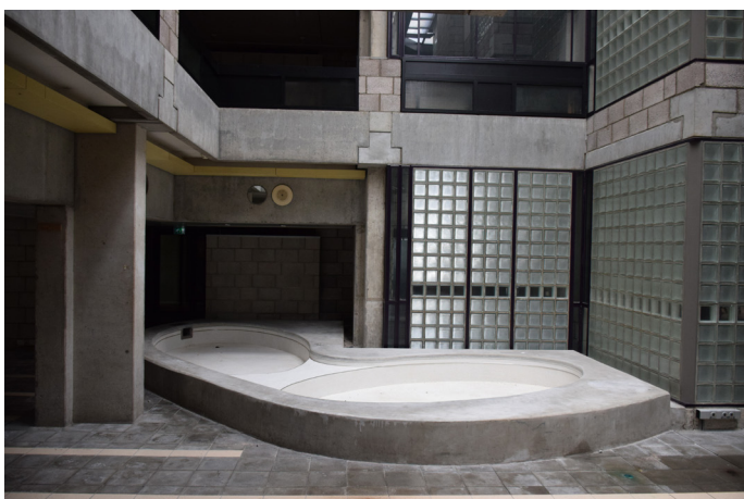
Fig. 186: Picture of the basin in the street.
