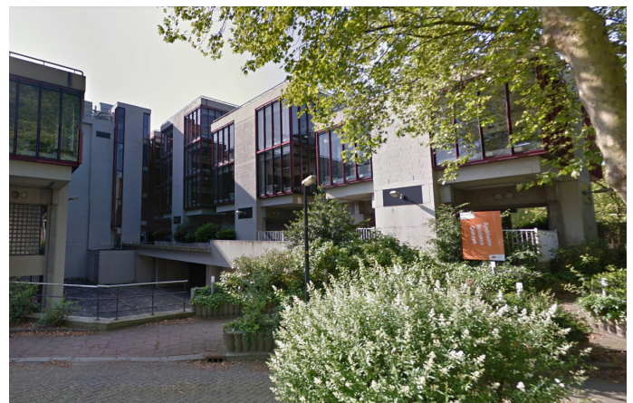
Fig. 16: North-west street enclosure.
