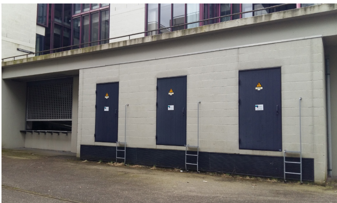
Fig. 156: Added technical room under bridge.
