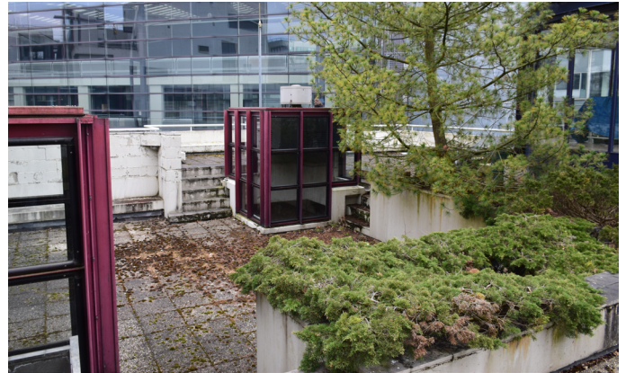
Fig. 135: Skylights and lowered terrace above the restaurant.
