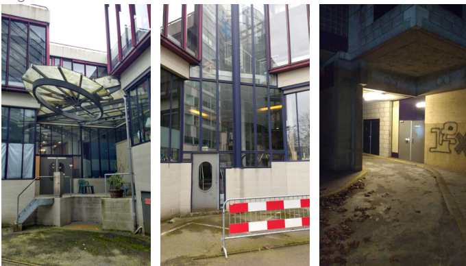
Fig. 21: Some of the secondary entrances.
