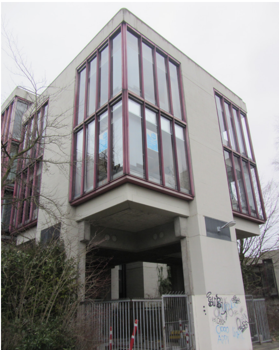
Fig. 59: Picture of the facade.
