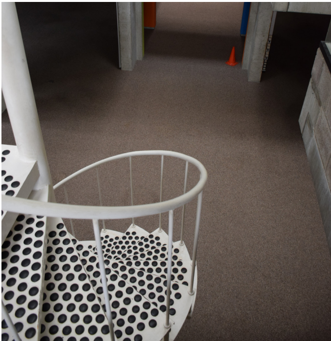
Fig. 170: Winding staircase as seen from above.
