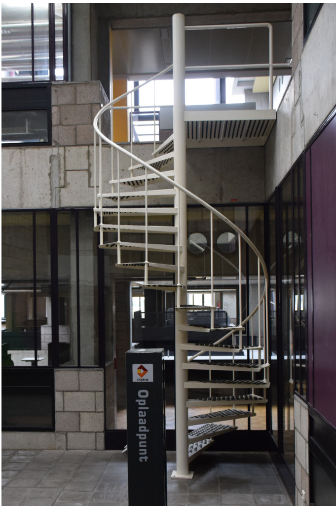
Fig. 171: Winding staircase as placed at several of the voids.
