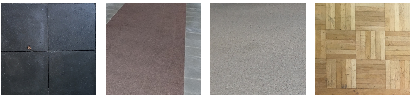
Fig. 54: Different materials as flooring are used to indicate zones, from left to right: paving stones, carpet in public street, carpet in offices, parquet.
