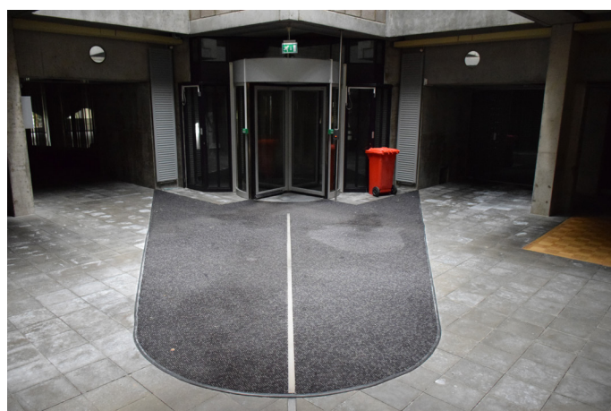
Fig. 206: Entrance from garage from the interior.
