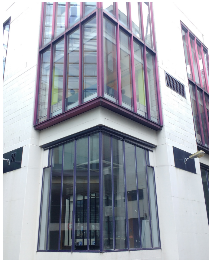
Fig. 201: Windows in front of and inbetween the construction.
