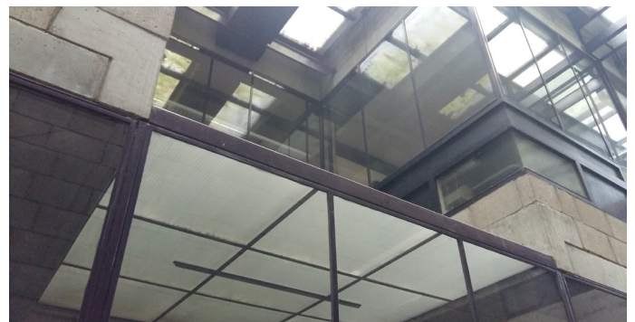
Fig. 149: Closed void between technical tower and computerroom.
