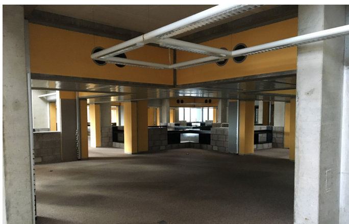
Fig. 63: Photograph of an empty office space in the abandoned building in 2018.
