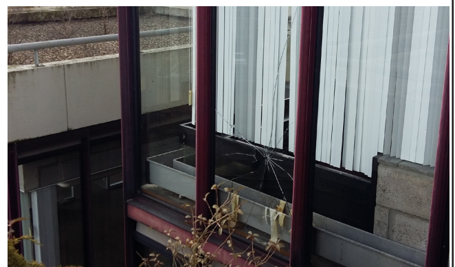
Fig. 32: Convectors behind the window.
