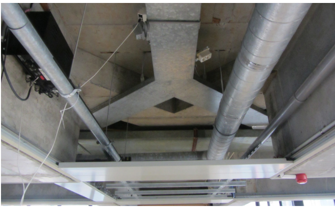
Fig. 130: Concrete cross supporting the primary beams.
