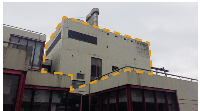
Fig. 209: The installation tower that can be used for orientation because of the way it stands out.
