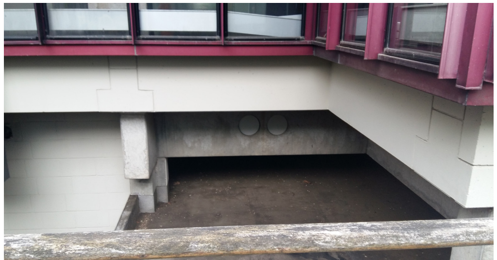
Fig. 214: Extra construction under computerroom for wooden floor.
