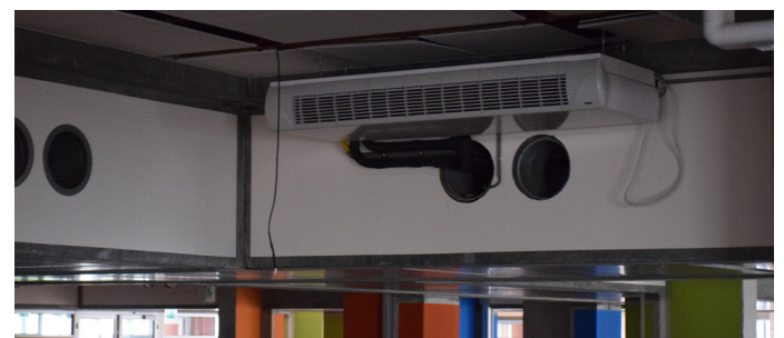
Fig. 40: Airco system added through the openings.
