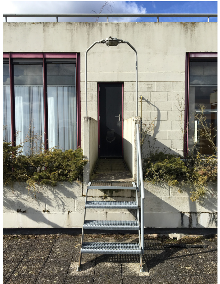
Fig. 69: Roof terrace entrance.
