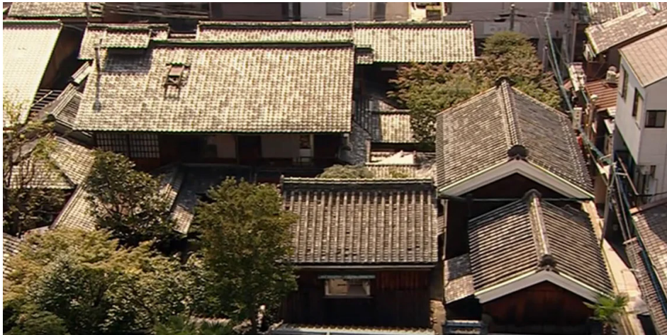
Fig. 1 – Top view of the buildings of the house of Sugimoto in Kyoto (Arte France, 2007)
