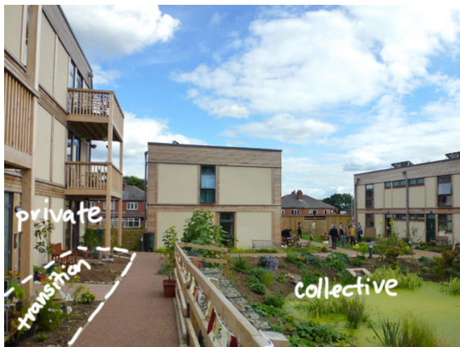
Fig. 89 - The low impact homes are made of timber and straw. Each home has a front garden looking out over the collective green spaces such as the pond (Modcell, 2021)
