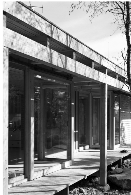
Fig. 68 - The facade on the side of the garden is almost completely made of openings with glass. Direct sun is prevented via the roofed veranda and via blinds. Views on different parts of the garden are given (Dextra Photo, n.d.)
