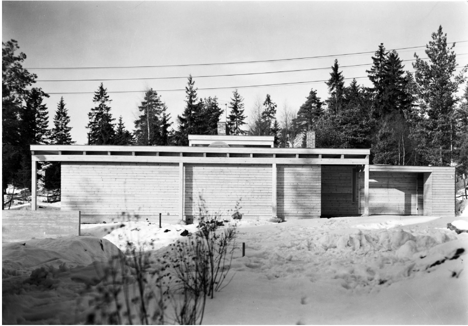
Fig. 63 - The facade facing the street is completely closed off with timber cladding. Passing by neighbours still are given a small idea of the way of living in the home via the beams and the posts that are shown. The beams show the one meter grid (Dextra Photo, n.d.)
