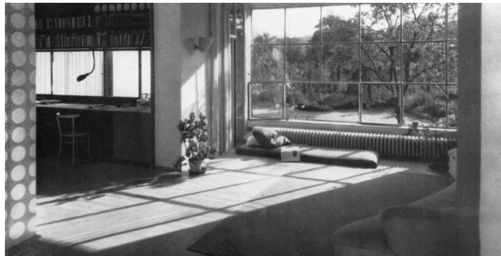
Fig. 10 - One is connected to the outdoors via a large multi-plane window with three horizontal layers: the top for daylight, the middle for a standing view and the bottom for the seated position (Elara Fritzenwalden, 1974)
