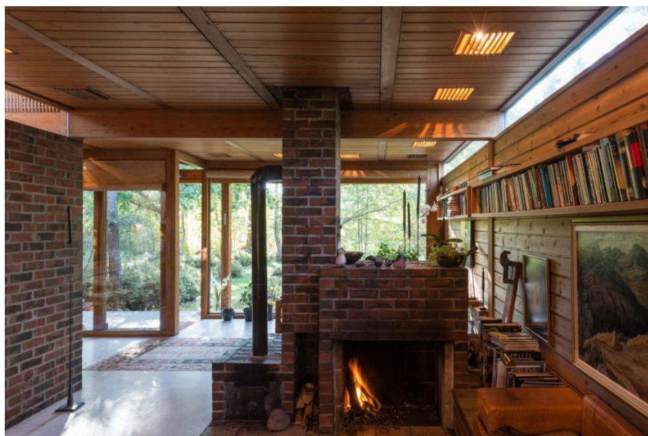
Fig. 58 - To allow natural light skylights are used in the kitchen and entrance area (on the top left). A hearth is placed next to the core in the living room (Berntsen, 2014)
