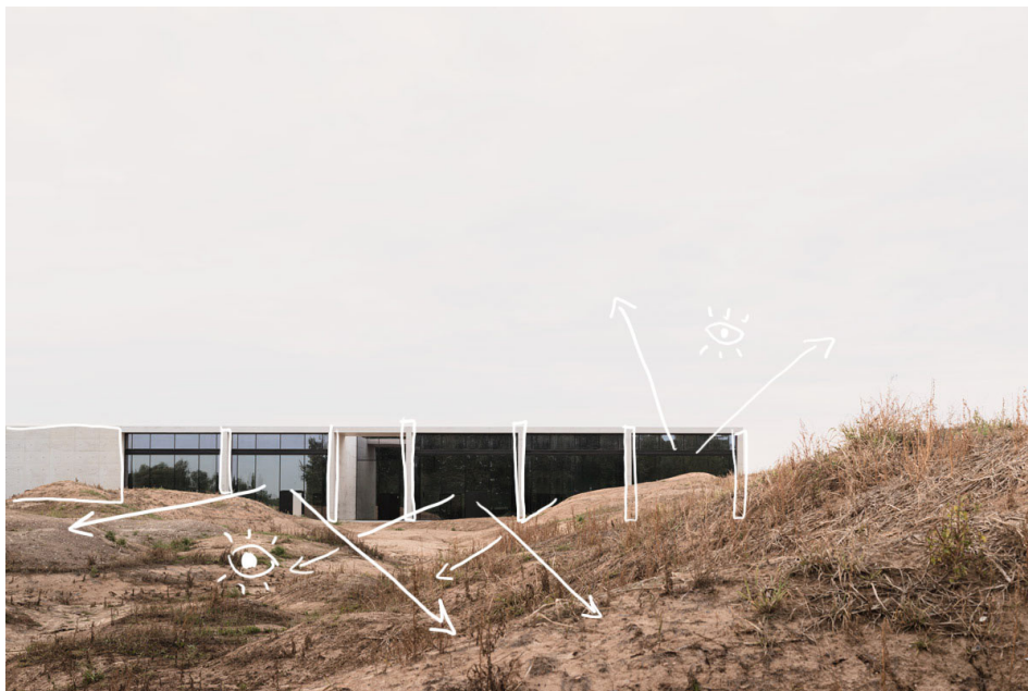
Fig. 39 - The building has a continuous shape within a hilly landscape. Large glazed walls allow wide views on the surroundings while its concrete walls in between allow for privacy (Bossi, 2018)
