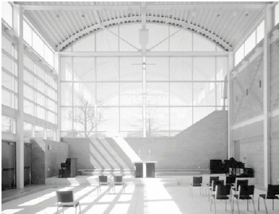
Fig. 90 - A mirror-glass cube with a steel vault resting on dusky-pink concrete blocks forms the sanctuary (Reatig, 2015)
