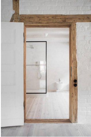
Fig. 31 - The door frames have been left untouched, showing the true nature of the timber frames. As a result the frame is not entirely straight (Hauck, 2019)
