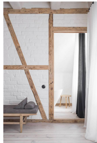
Fig. 36 - The framing of the bedroom walls are exposed to the eye and not covered by plaster (Hauck, 2019)
