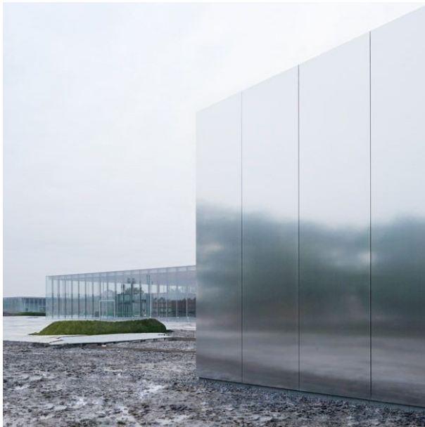
Reflective aluminium cladding
