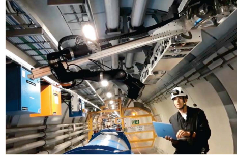
Fig. 2. Train Inspection Monorail (TIM) in the LHC tunnel.
