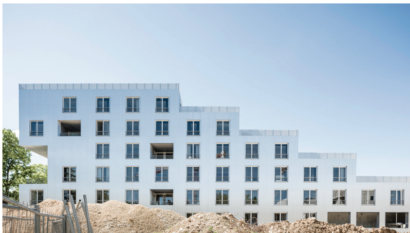
Fig. 19: Unite. From "Archdaily" by B. Verney, 2019 ( https://www.archdaily.com/929995/unite-s-experimental-housing-sophie-delhay-architecture/5df038f53312fdecff000192-unite-s-experimental-housing-sophie-delhay-architecture-photo?next_project=no ).
