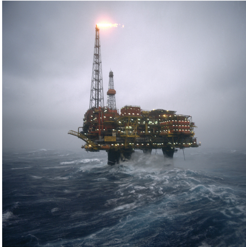
FIGURE 1.1. Shell Brent Charlie offshore structure in the North Sea experiencing loads by breaking waves [300].
