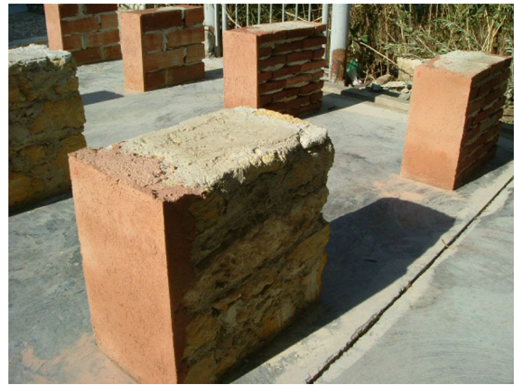
Fig. 8 Pilot application of crushed brick-air lime rendering mortar on wallettes constructed of stone (front row) and fired clay brick (back row) masonries
