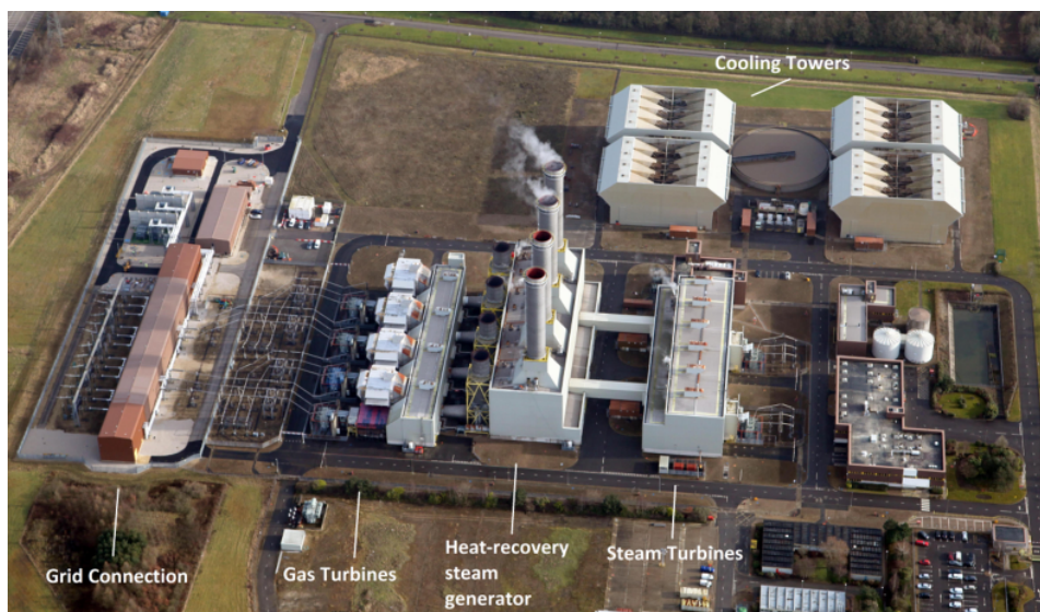
Figure 1.2: Uniper's Killingholme site before 2016 [2].
