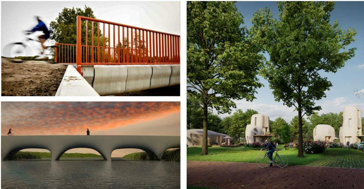
*Figure 1-4 The 3D printed reinforced concrete bridge in Gemert, North Brabant constructed in 201[39](left top). The 3D Printed concrete and parametric designed bridge will be placed in Nijmegen.[41] (left bottom).The world first commercial housing project based on 3D concrete printing in Eindhoven,2019 [40] (right).*
