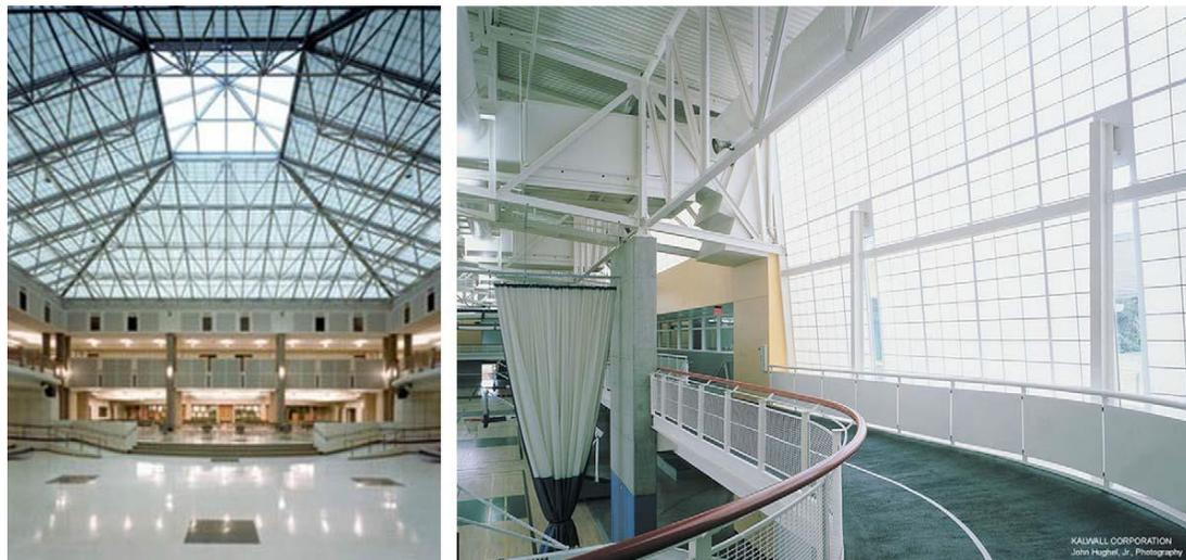
Figure 1-3 The utilization of monolith translucent aerogel insulation panels on the ceiling and facade as the high thermal insulation solution for the daylight purpose [11].
