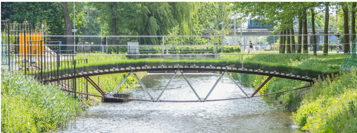
Figure 2.7: Picture of the Glass Truss Bridge located at the Delft University of Technology campus. The diagonals are made of bundled glass rods. The left-most and right-most diagonals are steel. The bridge has a span of 14 meters [1].
