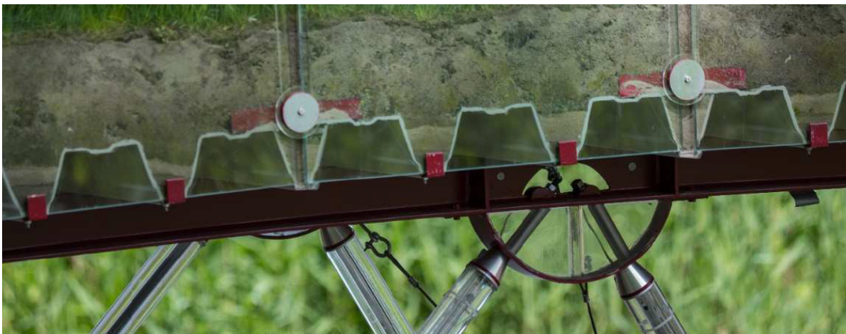
Figure A.5: A glass node in the bridge [1].
