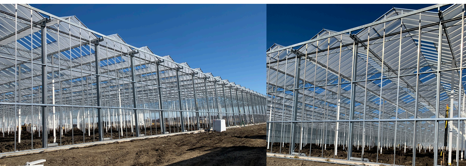
figure 8: MightyVine phase 3 under construction (VB, 2019)
