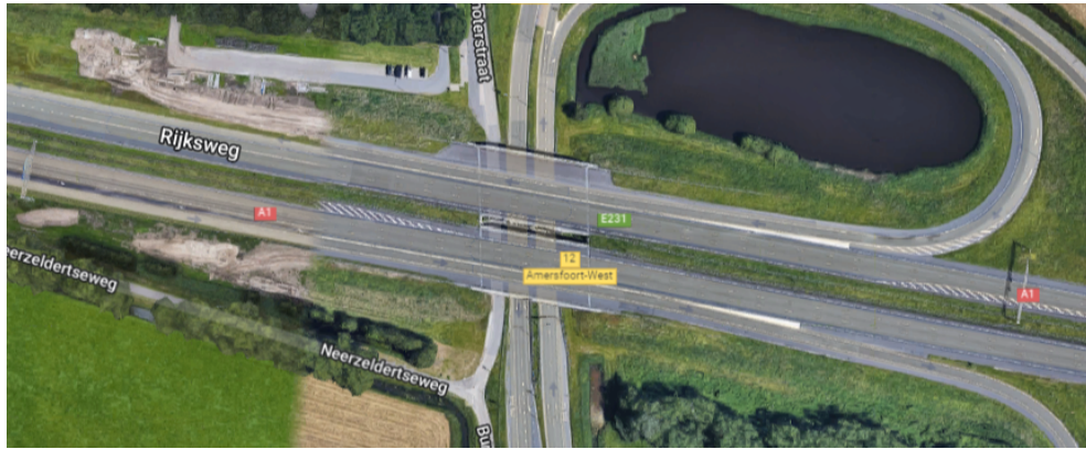
Figure 2.16: Overview of the new situation of the Zeldert viaduct, from [18].
