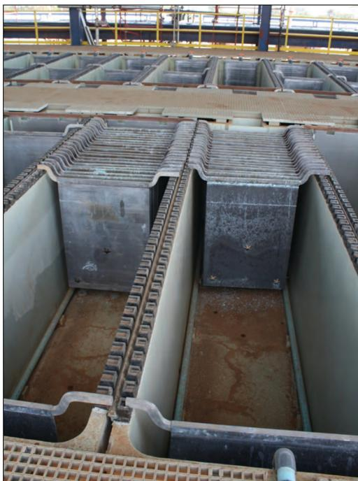
**Figure 3.5:** Lead anodes fitted in the electrochemical cells (Wimberley et al., 2011)
