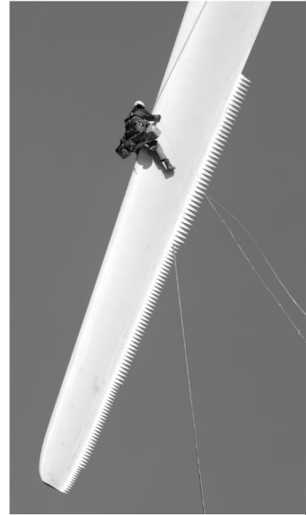
Figure 1-1: Climber removing trips from serrated blade
