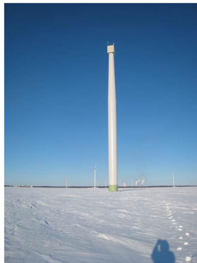
Figure 1. Test foundation with real static and dynamic properties of a complete 3 MW OWT installed to the northernmost part of the Gulf of Bothnia (Määttänen, 2010).
