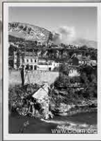
1994 Lučki most was destroyed
