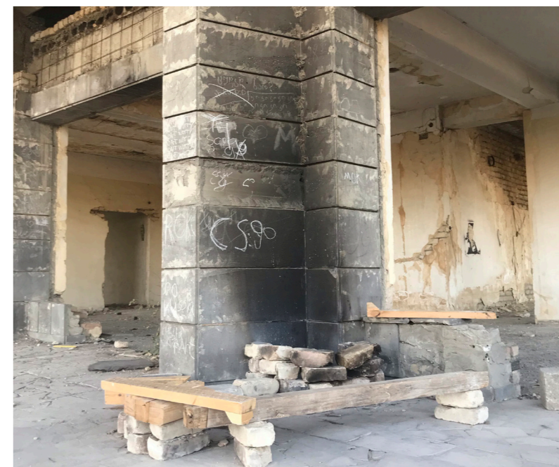
Figure 27_ A Year after the Inauguration of the Space
