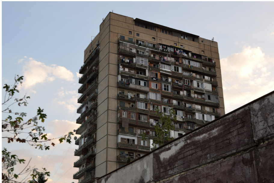
Figure 12_ Facade of the Dormitory Building
