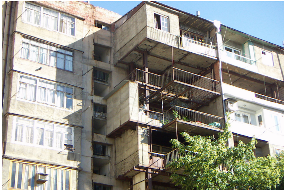
Figure 29_ Kamikaze Loggia Type 2 This documentation focused on typological differences between loggias. Photo, Sumbadze, G. c. 2000.
