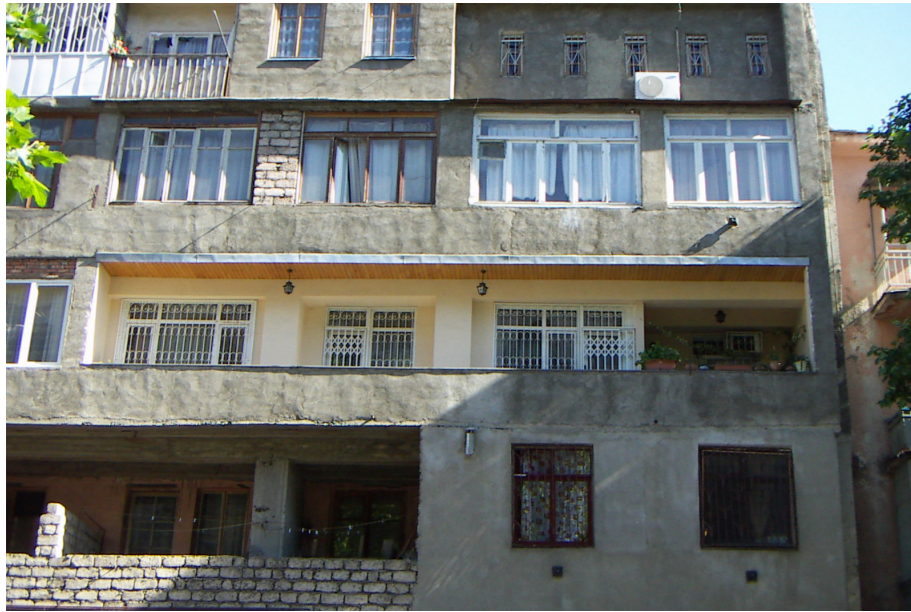
Figure 28_ Kamikaze Loggia Type 1 Documentation of Kamikaze Loggias by Gio Sumbadze. Photo, Sumbadze, G. c. 2000.
