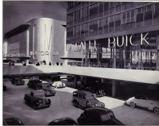
Figure 12 Separating pedestrian and motorised vehicles, creating separate entrances for buildings. Geddes, N. B. (1940). Magic Motorways (Vol. 1). Random House. https://openlibrary.org/books/OL7205622M/Magic_motorways .
