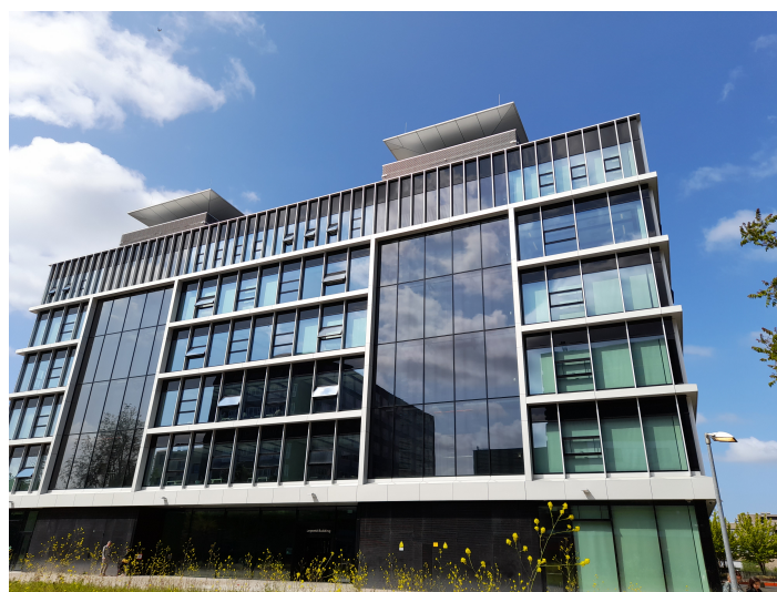
Figure 3: In the Langeveld building, a multipurpose study centre, at the Erasmus university in Rotterdam, a very low pressure hybrid ventilated building with solar/wind towers still has openable windows. The air can be cooled and humidified via a droplet shower in the central shafts, creating significant air pressure to induce the air flow [6,7].
