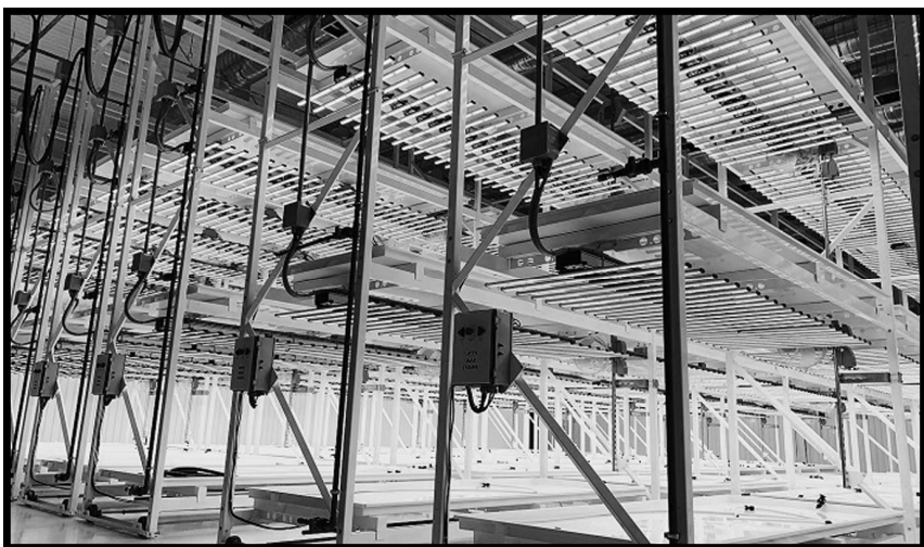
Fig. 24. Steel support structure for the hydroponic tray system. From RF Agriculture (2019).
