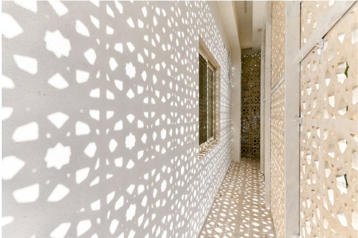
Figure 10: Example of a Mashrabiya, used to block direct sunlight 31
