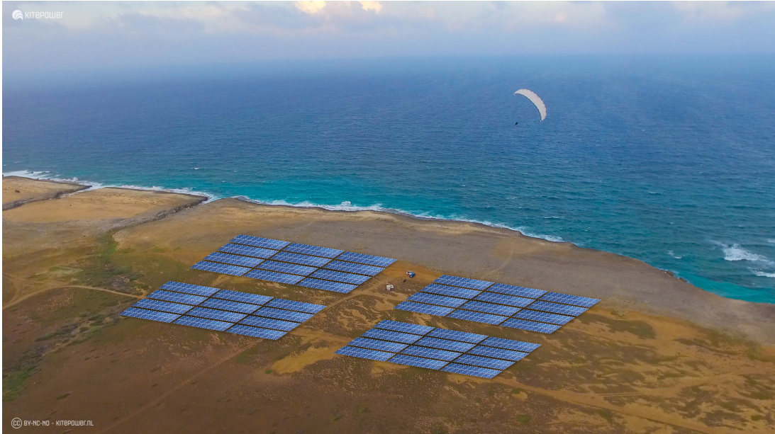
Figure 1.2: A photo composite of a HPP plant with solar PV and the Kitepower Falcon on a test site in Aruba [7].
