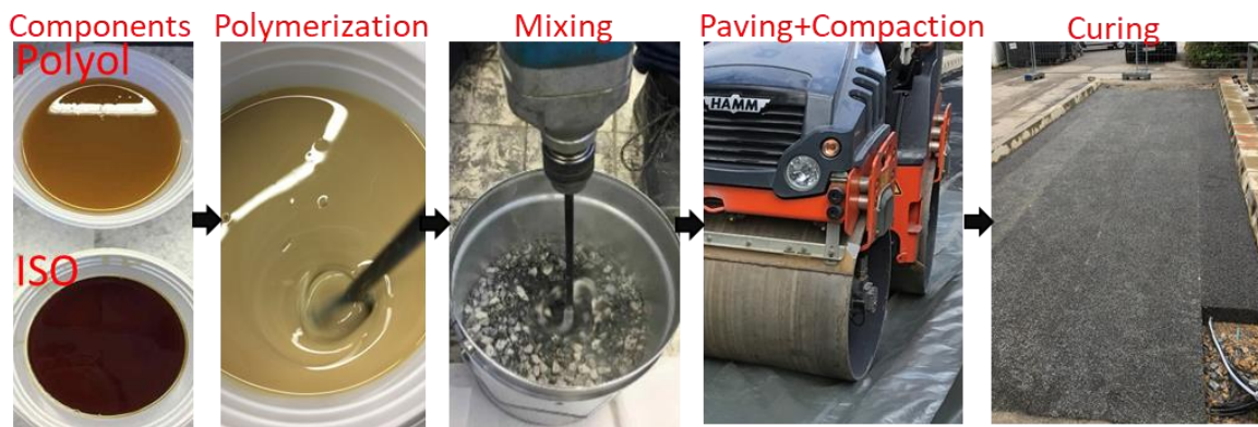
Figure 1. Production process of PUPM surface layer
