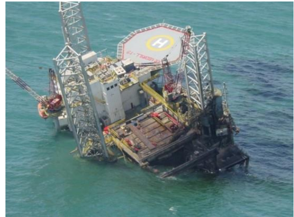
Figure 2.7 Photograph showing a jack-up failure due to a punch-through event in 2022 (Hunt and Marsh, 2004).
