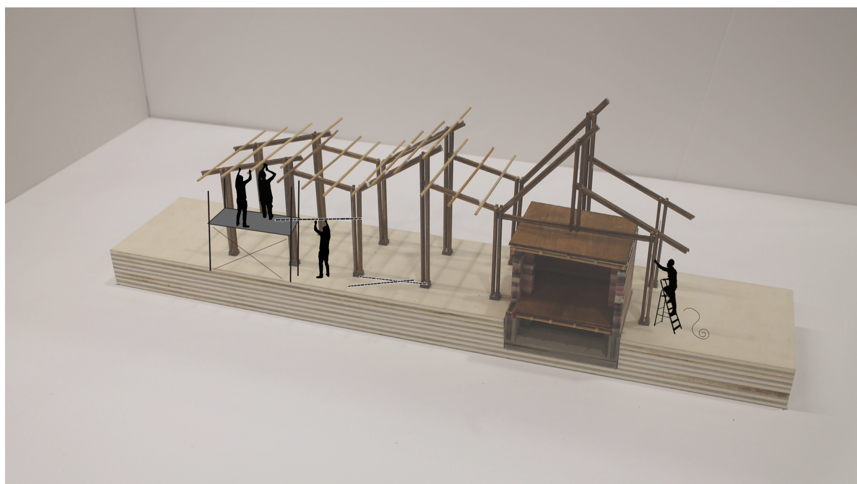
7. adding the bamboo purlins and rope bracing
