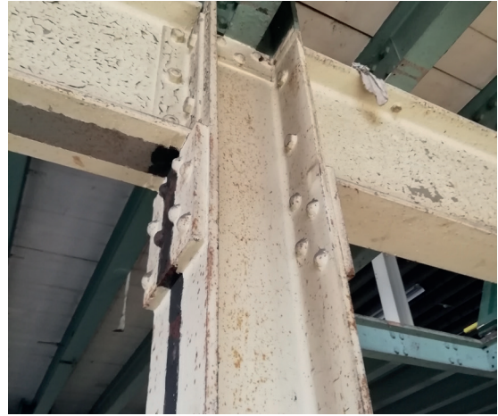
Figure 37: Visible construction Image by: Niels Steverink
