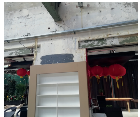
New openings with modern steel lintels run along the side connecting the Cathedral to the rest of the ensemble.
