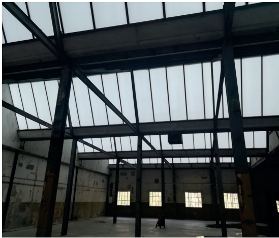
Figure 38: Visible construction Image by: Niels Steverink
