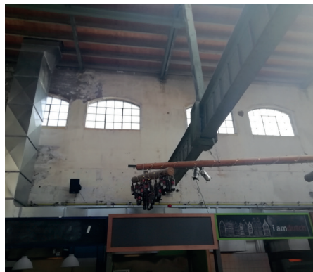
Two huge cast iron beams determine the look and feel of the lower section of the cathedral.
