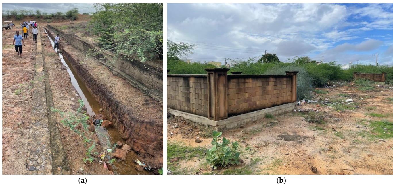
Figure 3. (a) A 500 m long drain discharges water from Umasar Lake toward the qanat system of 24 wells, of which two are depicted in image (b), to transport the water underneath a hill toward Hamirsar (authors 2022).
