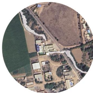
II encroachment - private company (tech)
