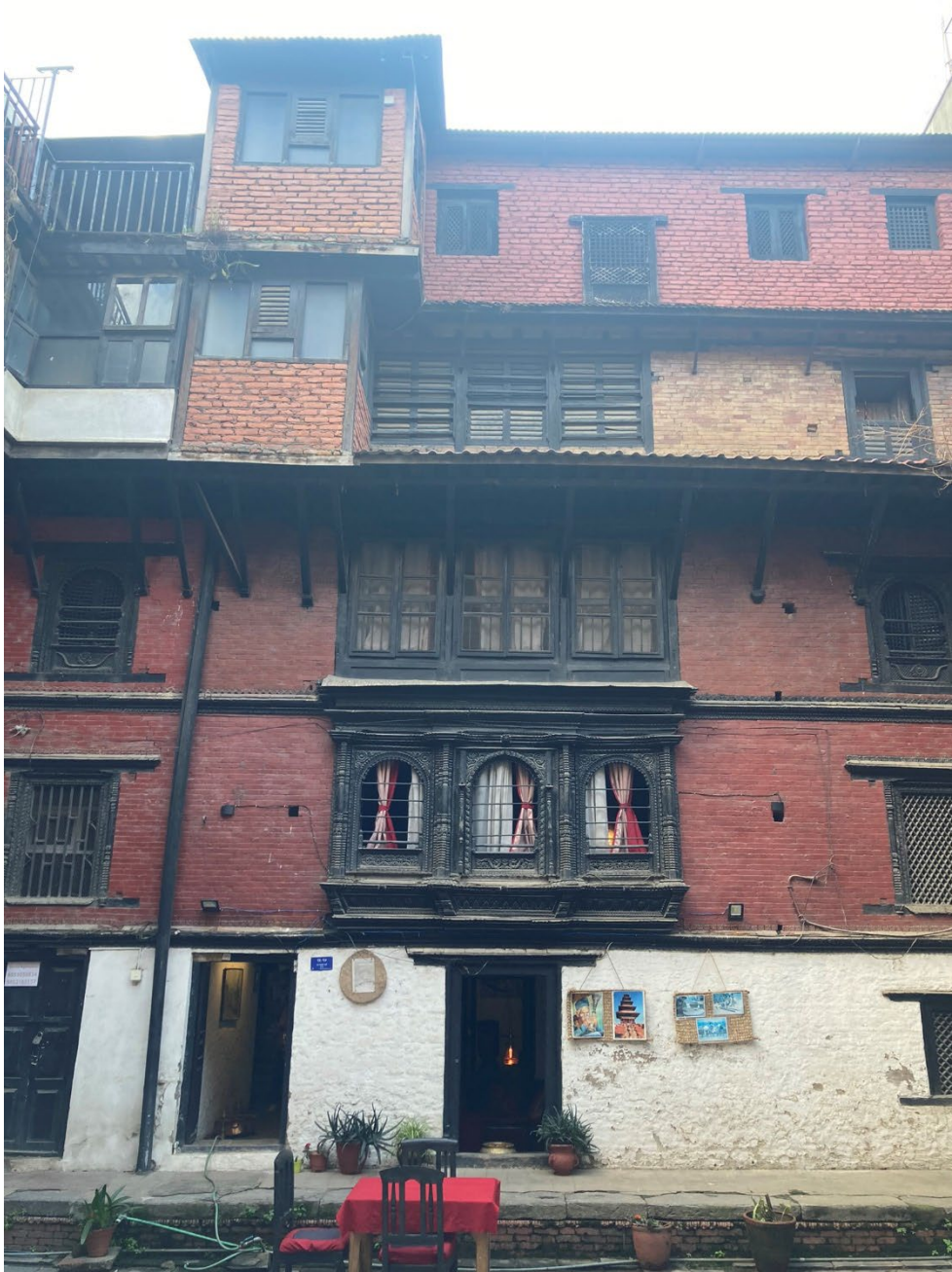
Figure 11: The approx. 300 year old Hira Guesthouse is a textbook example of a Newar house; embedded in a courtyard, originally 3-4 stories high, but topped up with another floor later on. The facades are made of fired bricks with mud mortar, of which the ground floor is plastered with lime. The 300-year age is a nuanced story though; parts could have been changed and reconstructed, which is not documented (Ranjitkar, 2023) (Author's own photograph, 2023)
