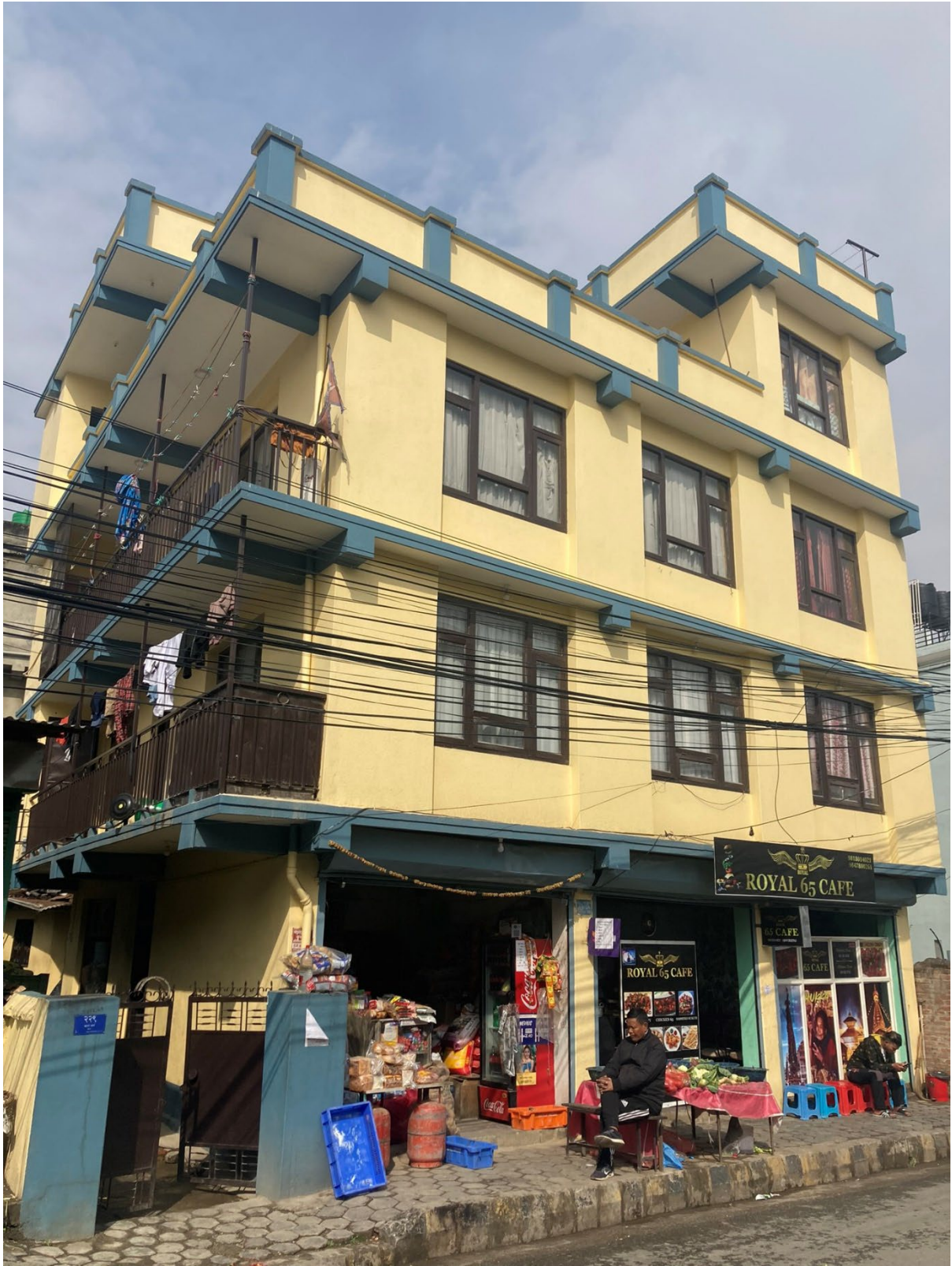
Figure 28: Typical modern concrete 'mushroom' housing, with a soft story on the ground floor containing a shop and a restaurant (Author's own photograph, 2023).
