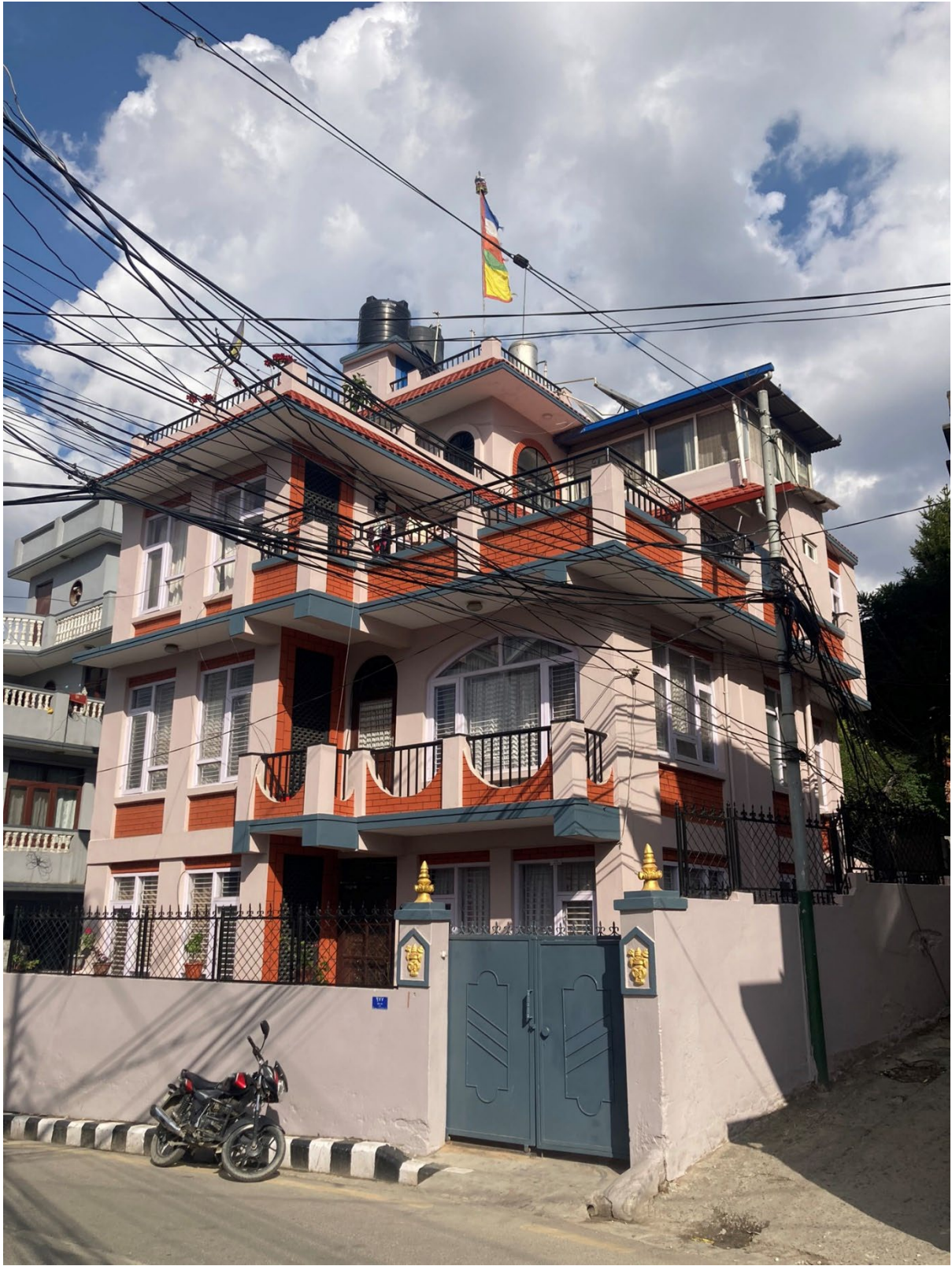
Figure 29: Similarly to figure 25; a concrete-framed and brick-infill house in Chakapat, Lalitpur.
