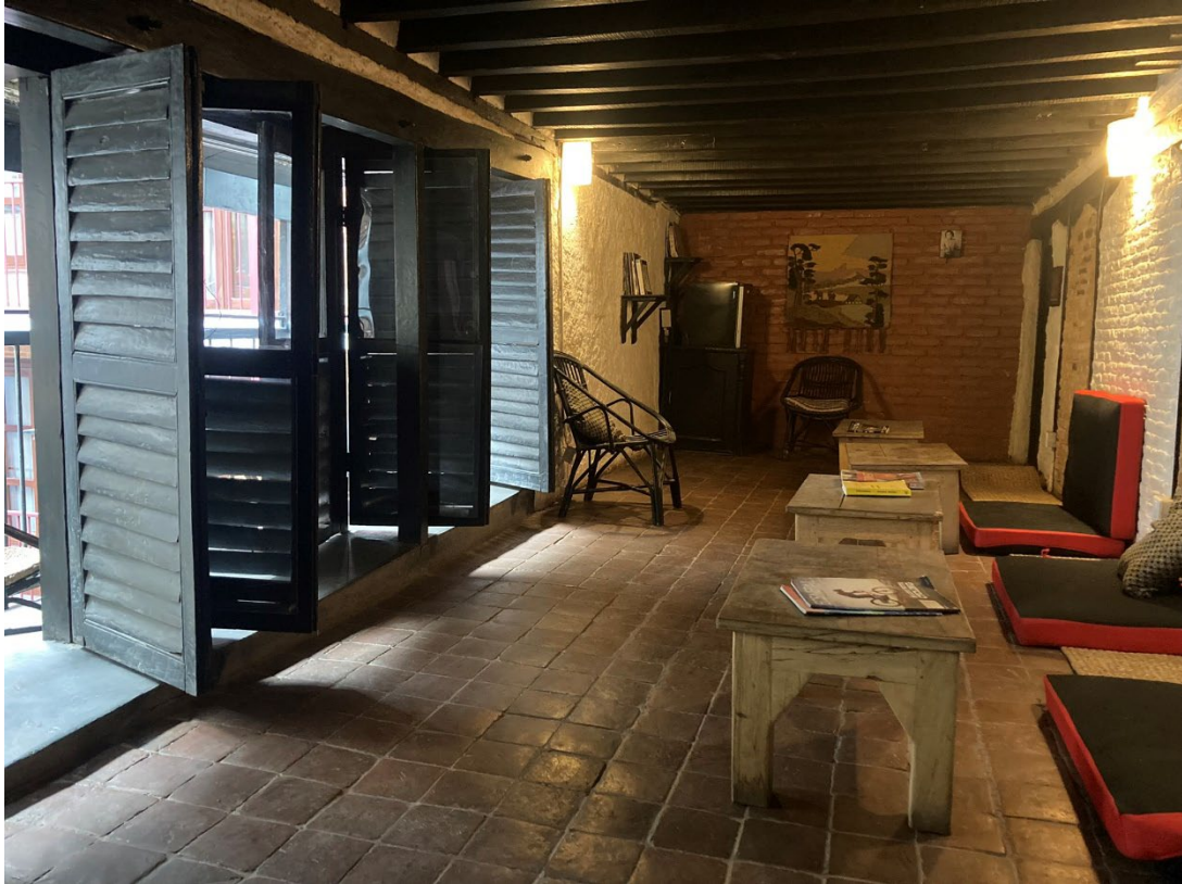
Figure 14: The inside of a typical Newar house, now transformed to a guesthouse living space. On the right, the dyā can be seen (white plastered wall). This 'spine' divides the 6-meter width in two spaces, therefore creating long and narrow rooms (Author's own photograph).
