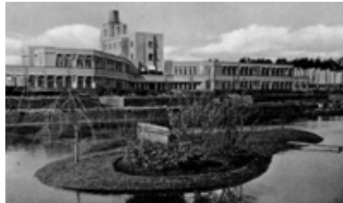
Sanatorium Noorder-Sanatorium, Drennoord
