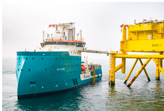
Figure 1.1: Acta Marine's Acta Auriga at BARD 1 preparing for crew transfer
