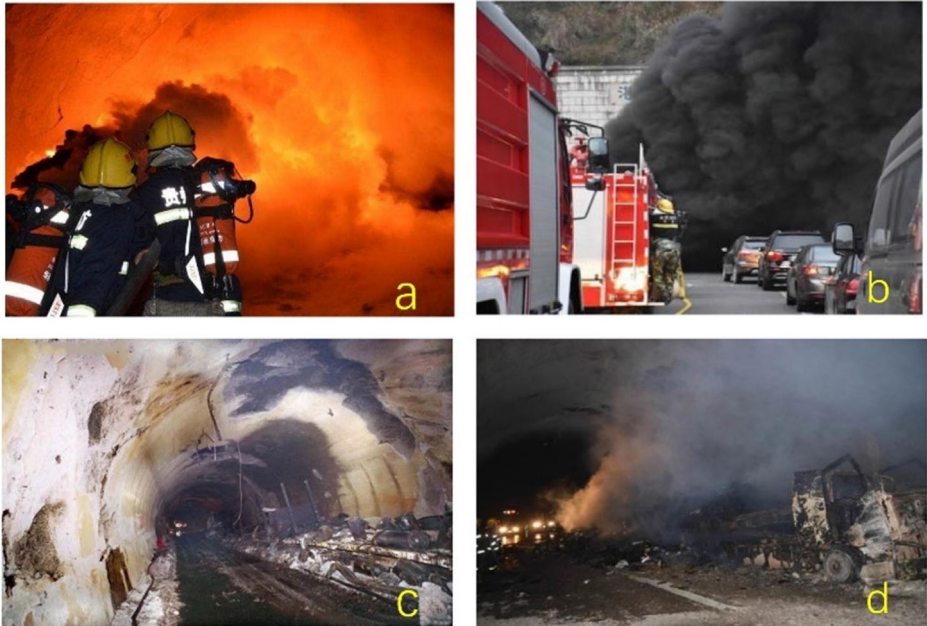
Figure 1. Major tunnel fire [18, 19].
