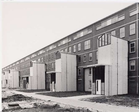
Figure 2. East side of the building with new staircases in front of the original back side of the building. From "Stadsarchief Amsterdam", by Archief van de Gemeentelijke Dienst Volkshuisvesting, n.d.
