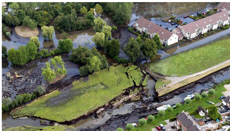
FIGURE 1.1: Sky image of the dike breach in Wilnis. (NOS, 2015)
