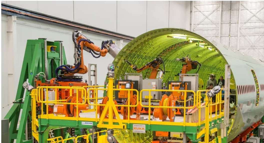
Figure 1-1: A pair of robots working on an airplane's fuselage in the Boeing FAUB project. [1]
