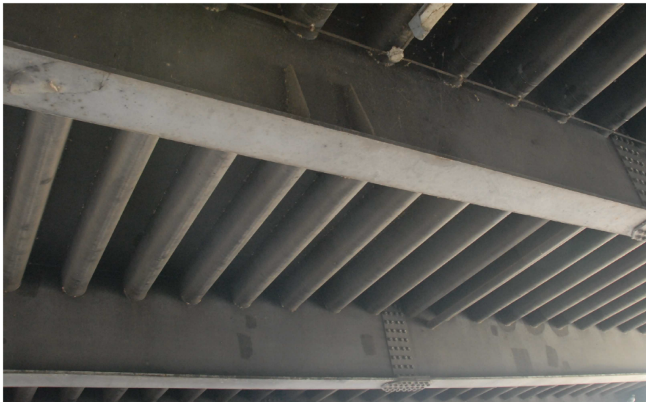
Figure 2.2: A part of the orthotropic deck as seen from the bottom.
