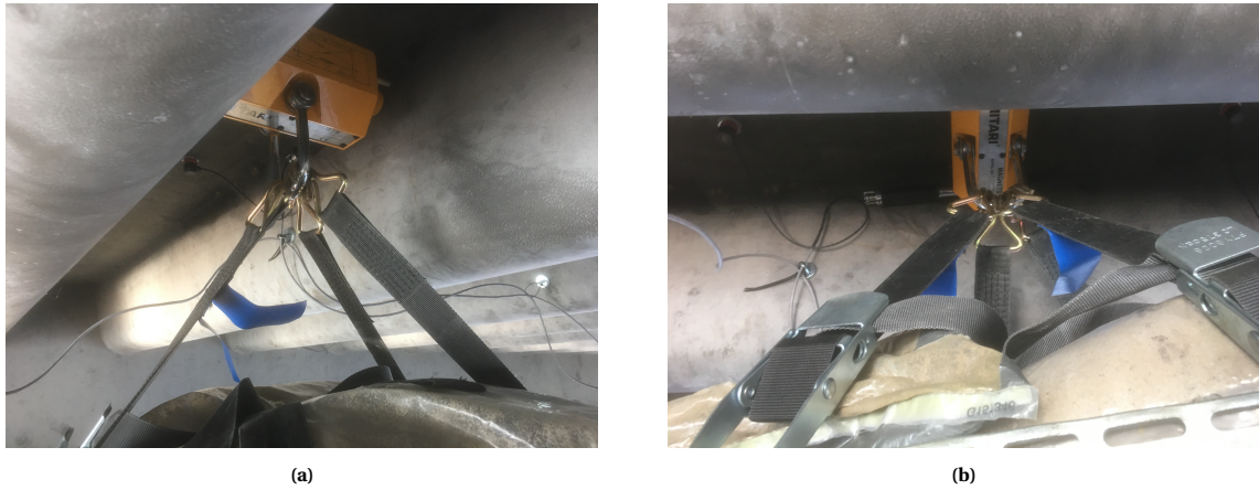
Figure 2.5: Attachment of added mass to bridge deck using a magnet.
