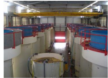
Drinking water pellet softening liquid-solid fluidisation
