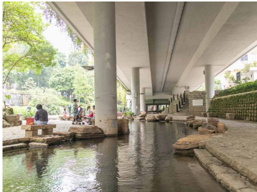
FIG. 4.5 Donghao Canal renovation / Source: Author
