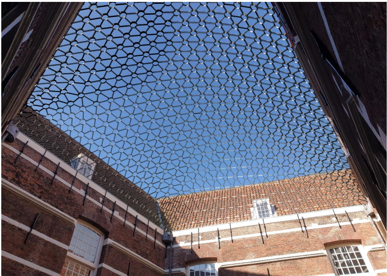
Fig. 13 Design for a cast glass shell structure covering the courtyard of the Armamentarium in Delft.
